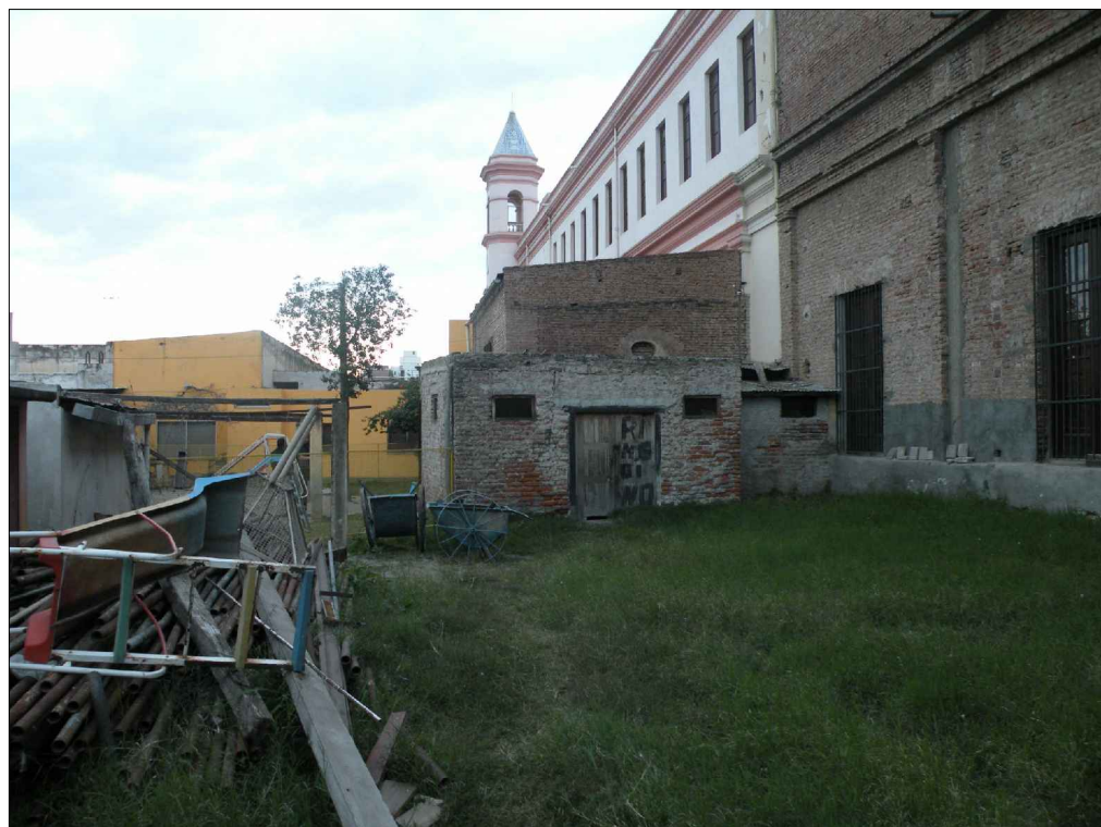
AREA A DEMOLER
